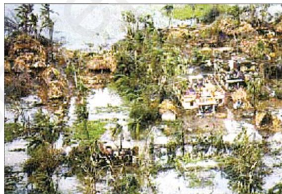
Destruction caused by a cyclone
